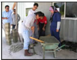
Concrete Slump Test
