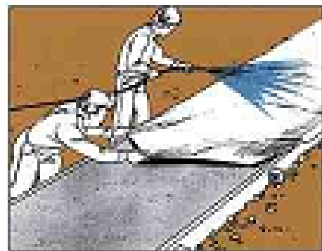
Water can be retained longer by using an absorptive cover.
